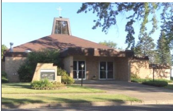
ST. LUKE'S CHURCH SANDSTONE, MN
