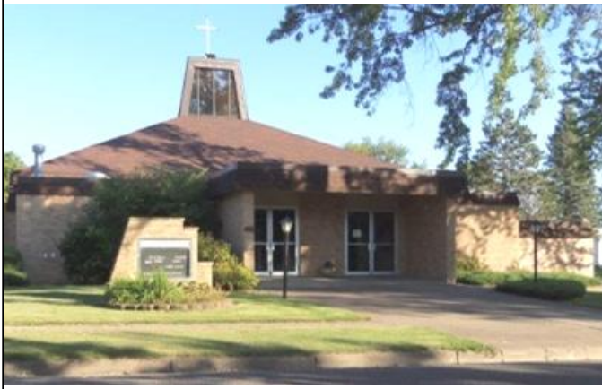
ST. LUKE'S CHURCH SANDSTONE, MN
