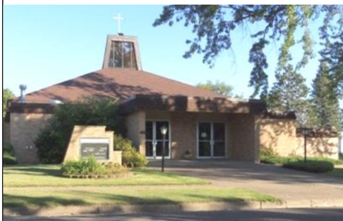
ST. LUKE'S CHURCH SANDSTONE, MN
