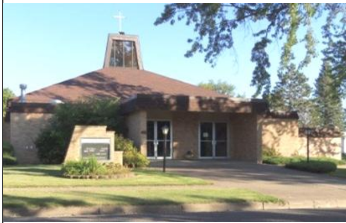
ST. LUKE'S CHURCH SANDSTONE, MN
